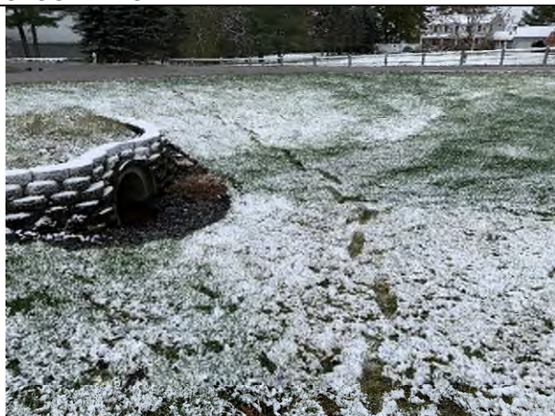
29 Gundalow - 1 (Drainage Area)
