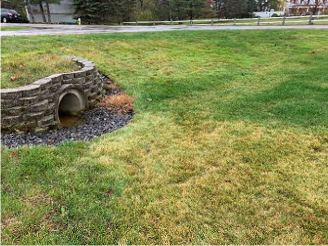
29 Gundalow - 1 (Drainage Area)
