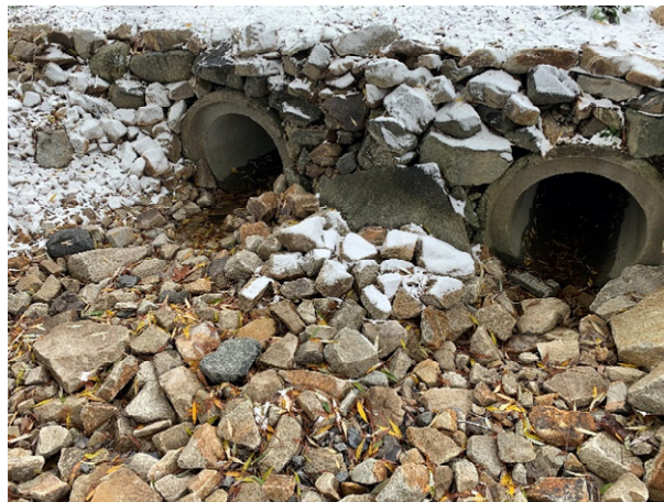
64 Gundalow - 2 (Drainage Course)
