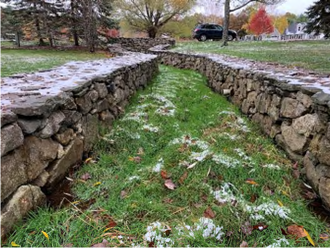
4 Brickyard – 2 (Drainage Area) facing northeast
