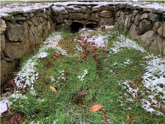
4 Brickyard – 3 (Drainage Area) facing southwest
