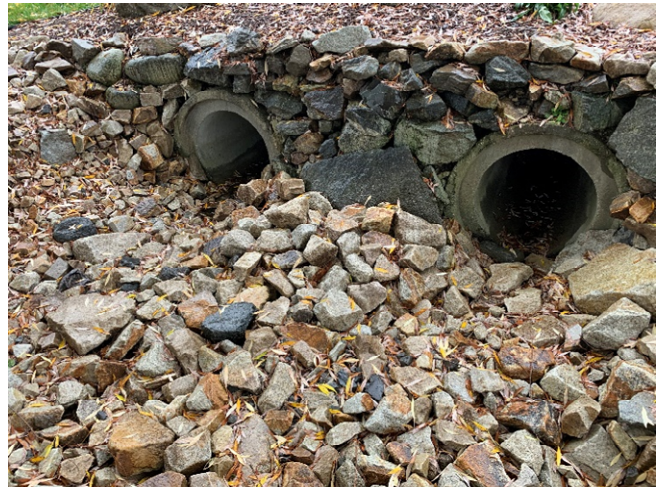
64 Gundalow - 2 (Drainage Course)
