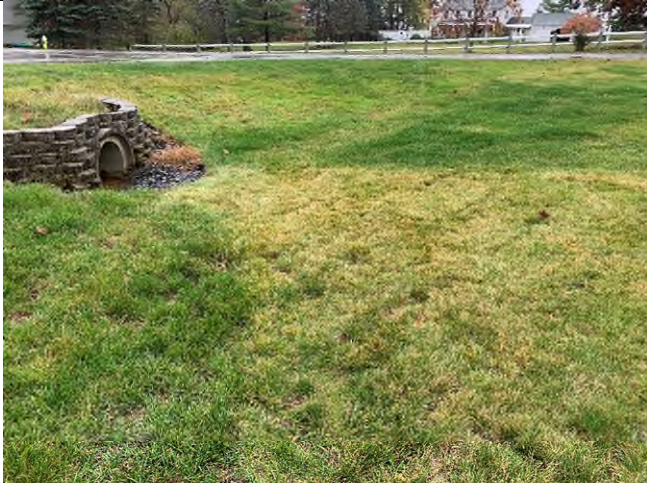
29 Gundalow - 1 (Drainage Area)
