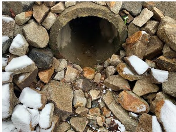
64 Gundalow - 1 (Drainage Course)
